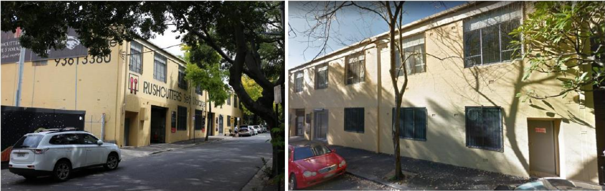
Figure 3: Photographs of the site and existing building, looking south (left) and looking north-east (right)
