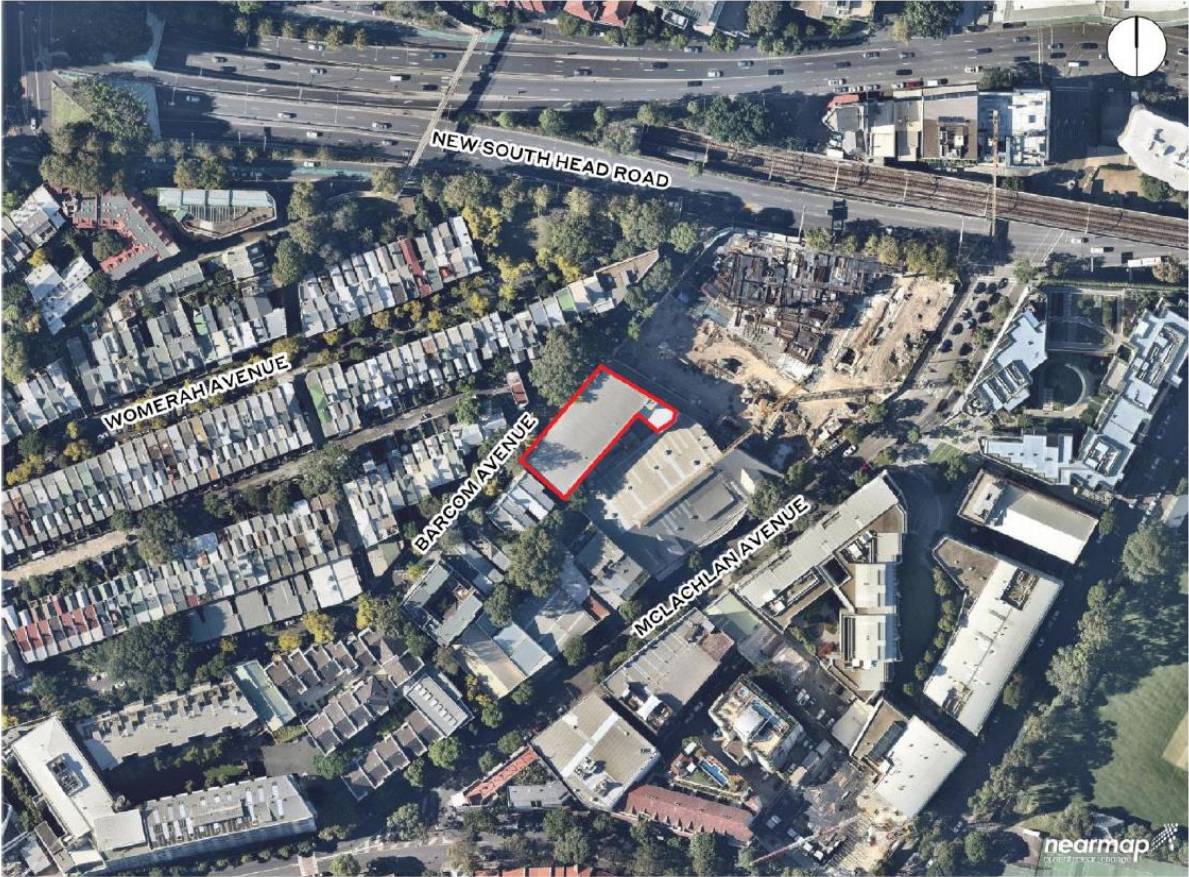
32-60 Barcom Avenue (the site)
